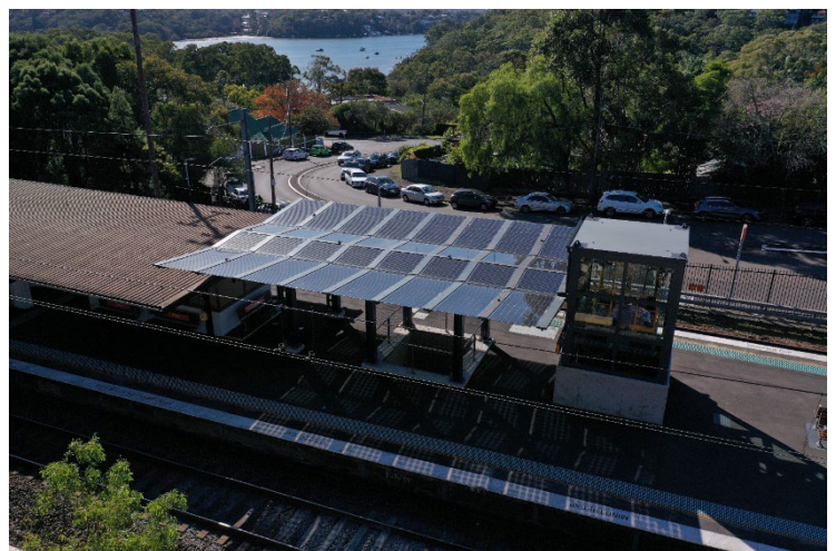
Como Train Station, in Sydney's Sutherland Shire, is now powered with solar energy via an innovative Solar Photovoltaic Glass canopy, a first on any NSW rail network. Credit: TfNSW
