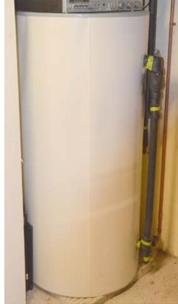
The pipework around the tank is fully insulated. To further increase efficiencies, all the hot water pipes to taps and showers have also been insulated.
